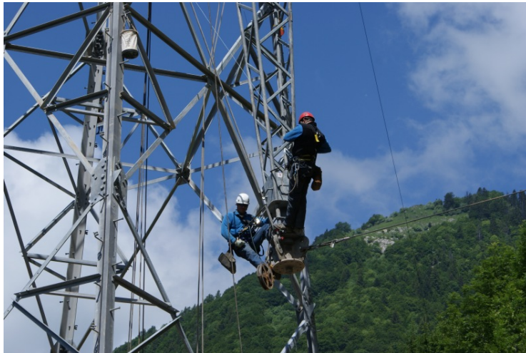
Figure 1: A maintenance team performing an intervention on overhead power lines
